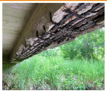
Existing bridge built in 1966. Concrete tee-beams are reaching the end of their service life.
