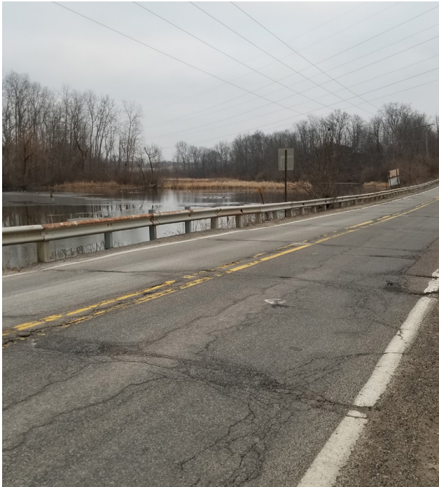
The Saline-Milan Road Bridge will be replaced this summer
