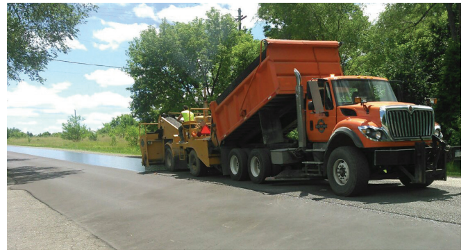
Crews chip sealing on Pontiac Trail
