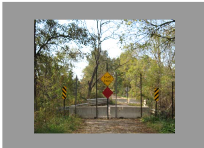
Above is an example of one of five closed bridges in the County. With no eligible funding source available to replace the bridges, the Road Commission was forced to close the bridges due to their unsafe condition.
